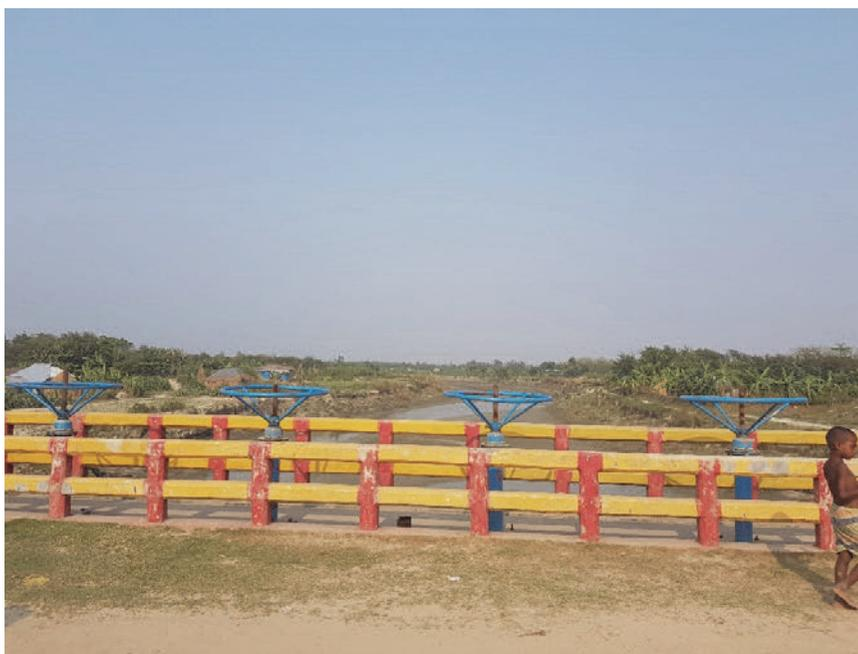
**Fig. 6.3.** Lift gate operating deck at C/S of Sluice DS-1, Char Nangulia.
