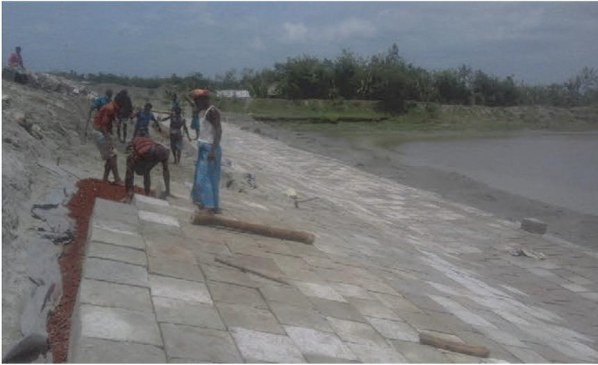
**Fig. 6.2.** Construction of Caring khal closure, Char Nangulia.
