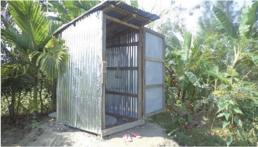
**Fig. 6.8.** Single pit latrine, where the super-structure is built by the stakeholder and the sub-structure by DPHE, Noler Char.
